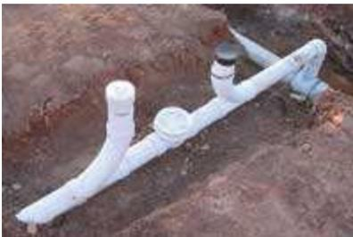
A backflow valve can stop sewage from backing up into your home. Clean it periodically to keep it working.
